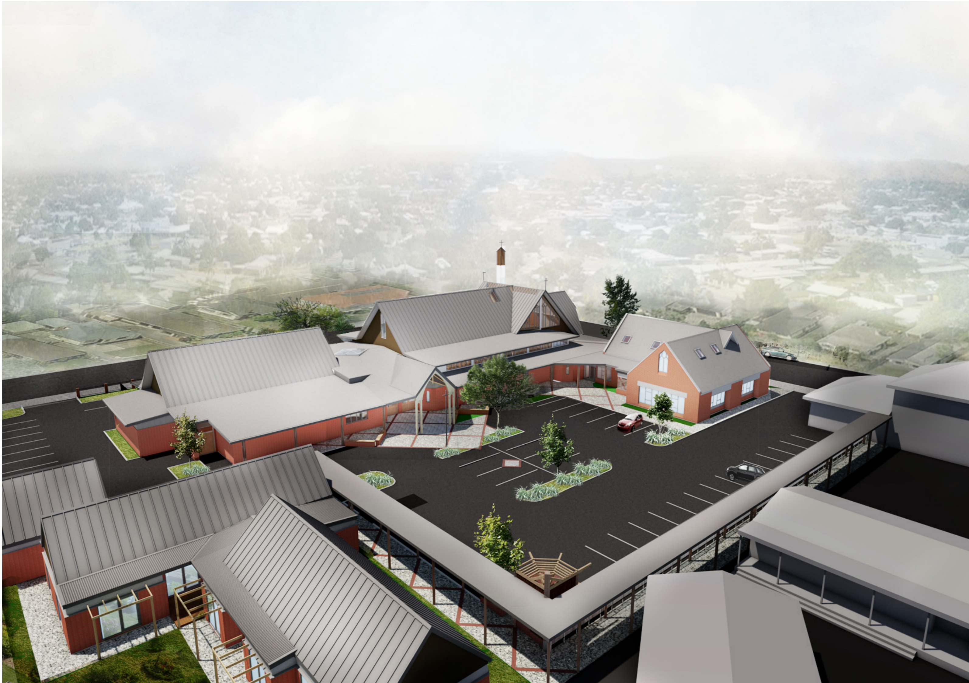
Overview of the Community Courtyard, Presbytery, Pastoral Assembly, Main Church and Pastoral Centre, with St Josephs School in the right.
